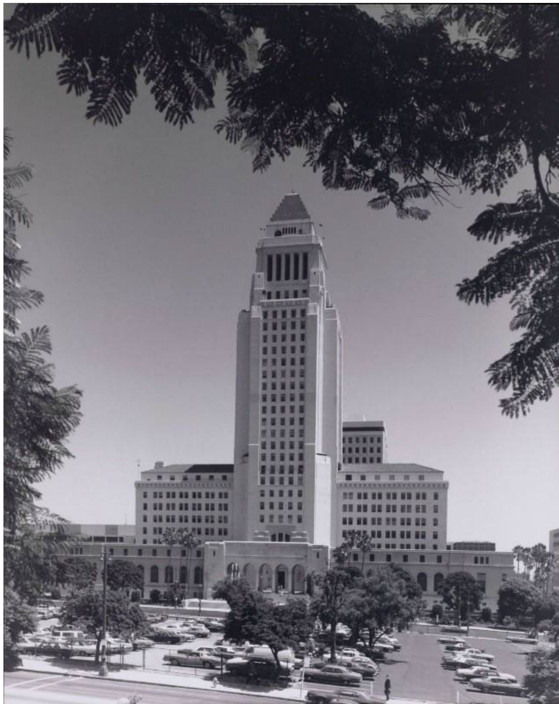
Figure 12 Los Angeles City Hall, photographed by Julius Schulman, view east, 1978. © J. Paul Getty Trust. Getty Research Institute, Los Angeles (2004.R.10).
